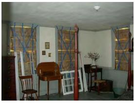
First floor south room at Thompson House with sashes removed and temporary insulation installed.
